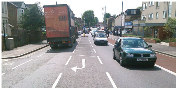
Road features, such as right-turn pockets laid out with wide central hatching, are often unnecessary
